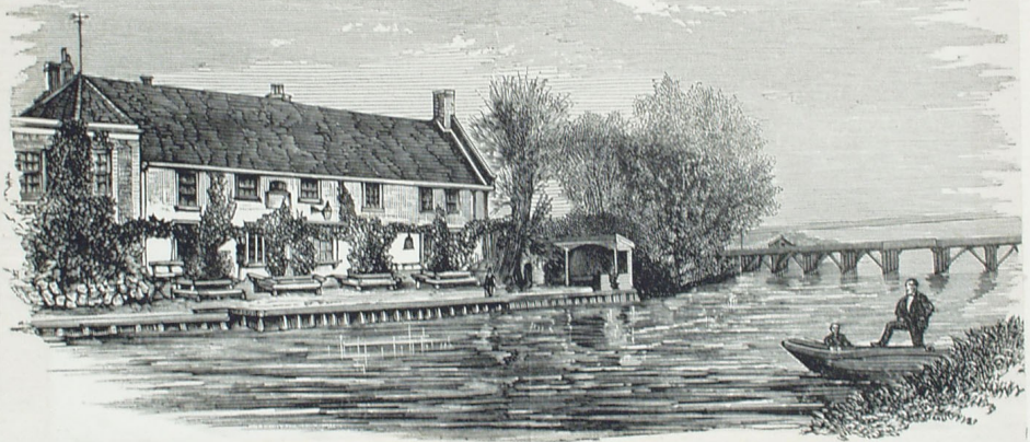
THORPE GARDENS, WITH THE FATAL RAILWAY BRIDGE AND FIELD'S BOAT-HOUSE IN THE DISTANCE.
