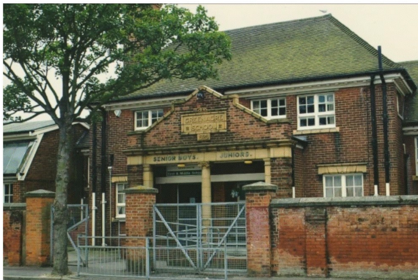
The Greenacre School on Dickens Avenue in Great Yarmouth
